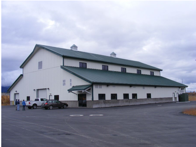
Cascade, ID WWTP
