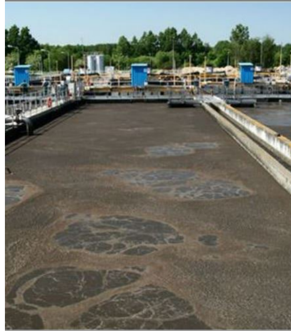
A wastewater plant with outside basins
